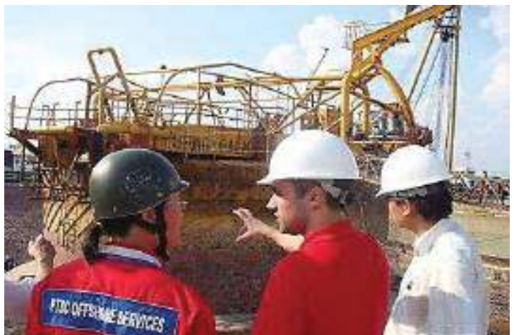
PAINTING A REFURBISHED MOORING BOUY
