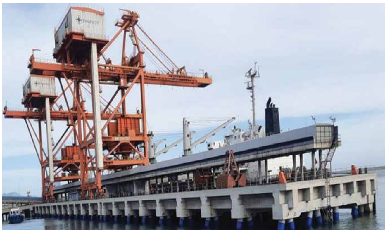
PROTECTED JETTY PILES
