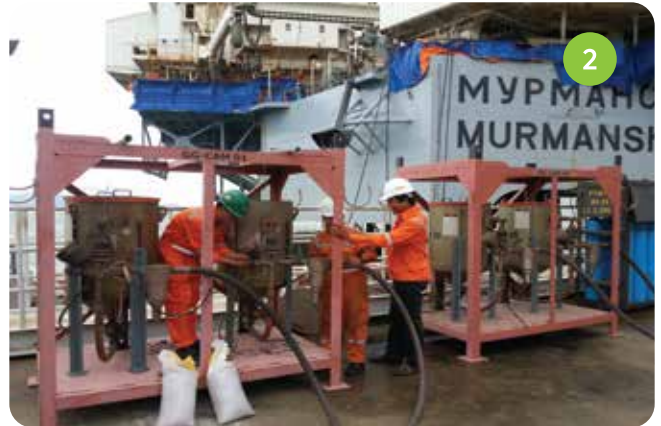
1 Blasting water-encapsulated abrasives
