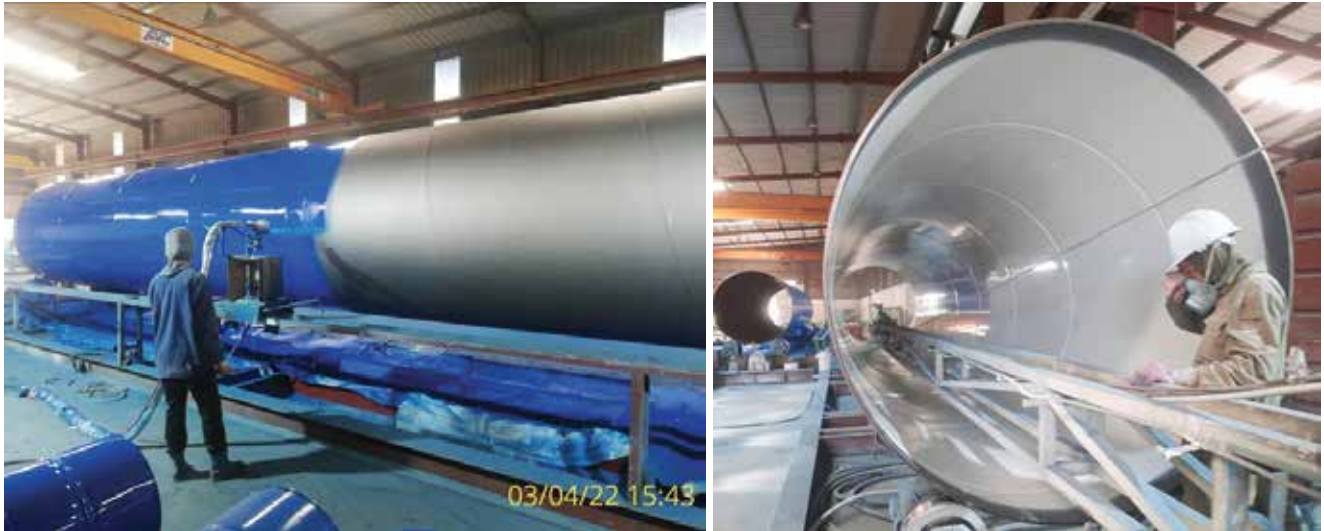
APPLYING PAINT INTERIOR AND EXTERIOR PIPE
