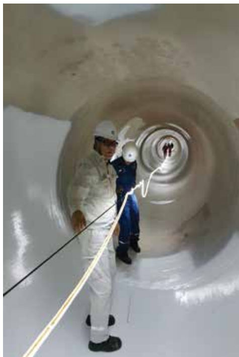
PAINTING INSIDE A SEAWATER PIPELINE OF DUNG QUAT REFINERY
