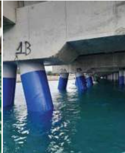
PROTECTING THE JETTY PILES OF VINH TAN POWER PLANT
