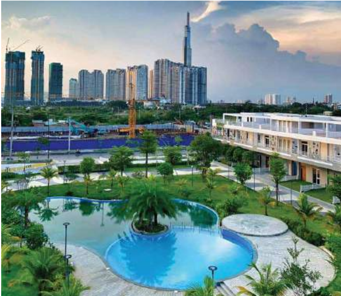
PAINTED THE LAKE VIEW APARTMENT – DIST. 2, HCMC
