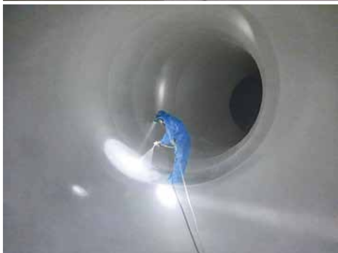
PAINTED THE INSIDE OF SEAWATER PIPELINE – VUNG ANG THERMAL POWER PLANT
