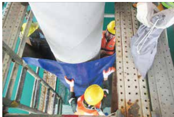
WRAPPING THE JETTY WITH 250UHD
