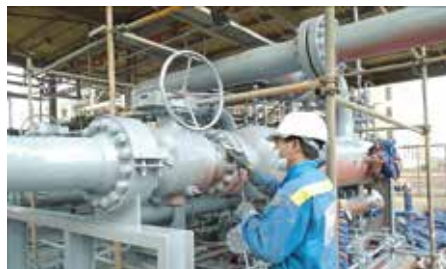
GAS PIPELINES PAINTING
