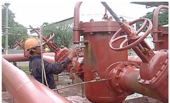
PAINTING THE GAS SEPARATION STATION OF PHU MY
