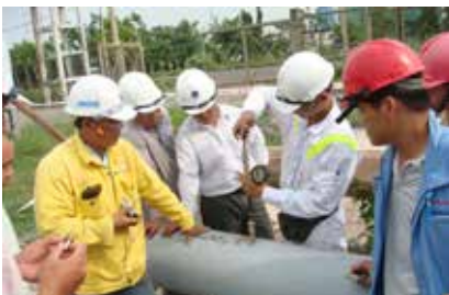
PULL OFF CHECKING
