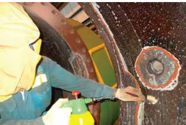
REPAIR THE HOLE INSIDE THE CONDENSER
