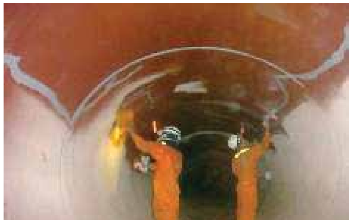
PAINTING INSIDE THE PIPELINE – PHU MY
