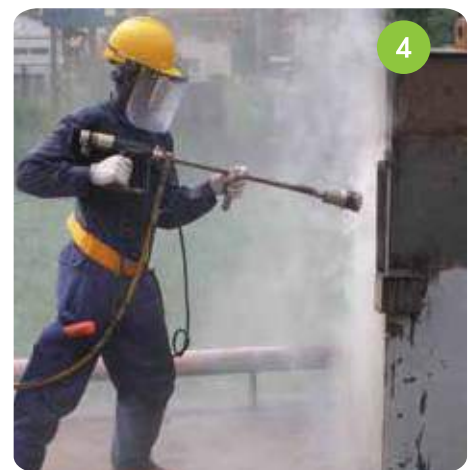
2 Dry abrasive blasting
