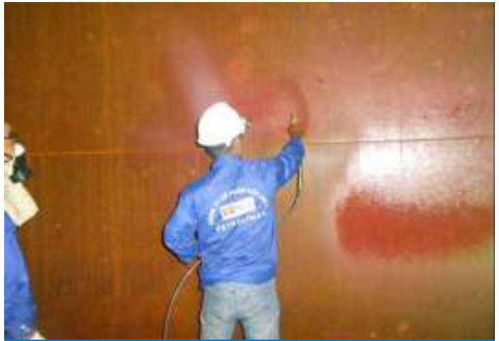
APPLYING THE 1 ST COAT
