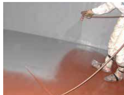
PAINTING INSIDE THE TANK
