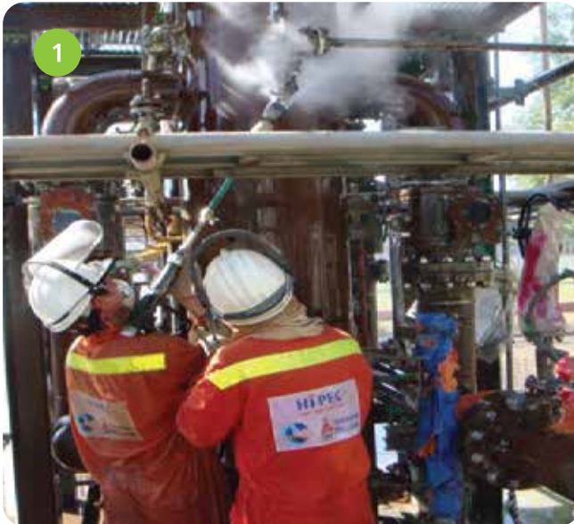
3 Blasting using CO 2
