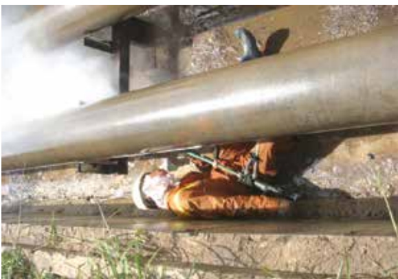
ULTRA-HIGH-PRESSURE WATERJETTING OF ONLINE GAS PIPELINES
