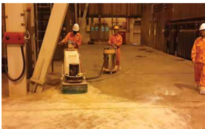
GRINDING – VACUUM CLEANER
