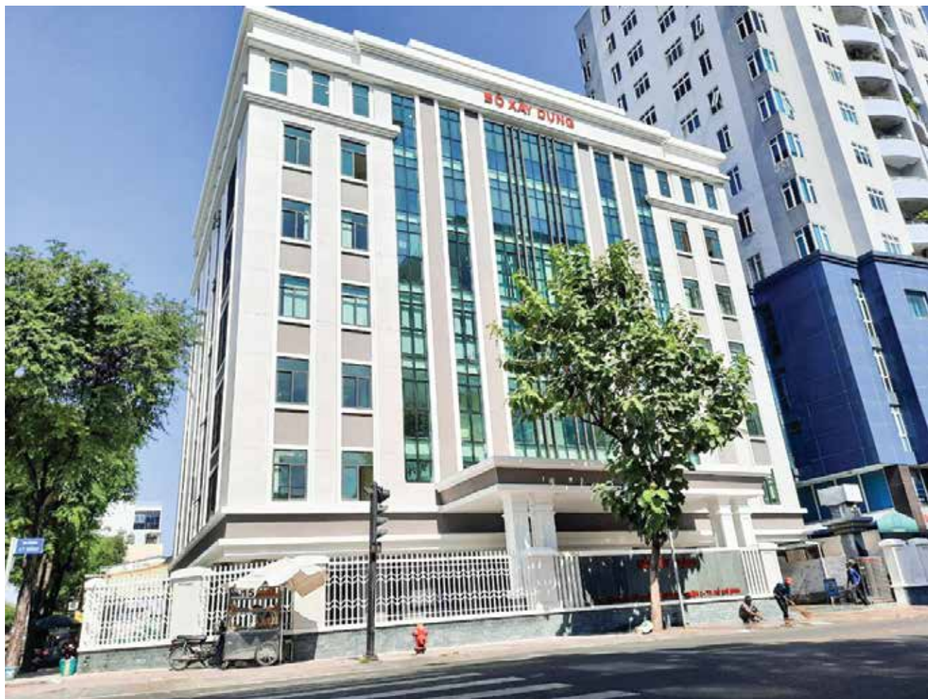
PAINTED THE SOUTHERN OFFICE – MINISTRY OF CONSTRUCTION
