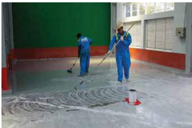
2 ND COAT APPLICATION
