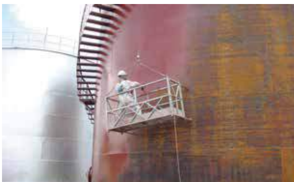
PAINTING OIL STORAGE TANK
