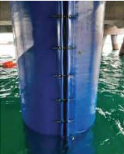
PROTECTING THE JETTY PILES OF VINH TAN POWER PLANT
