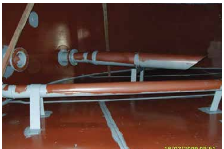
PAINTING INSIDE JET A1 FUEL TANK
