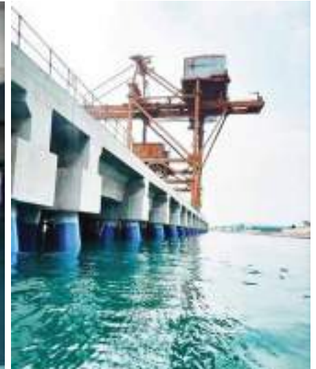
PROTECTING THE JETTY PILES OF VINH TAN POWER PLANT
