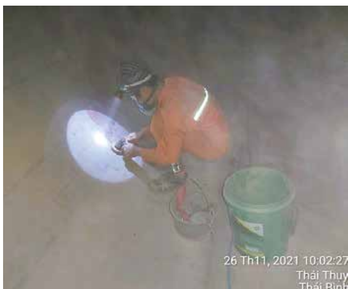
PAINTED THE INSIDE OF SEAWATER PIPELINE – THAI BINH THERMAL POWER PLANT
