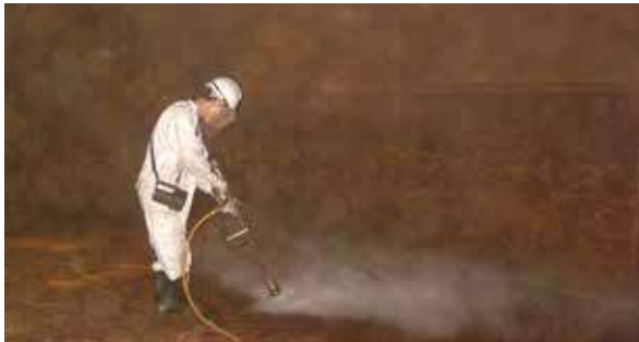
SURFACE PREPARATION OF TANK BOTTOM BY ULTRA-HIGH PRESSURE WATERJET
