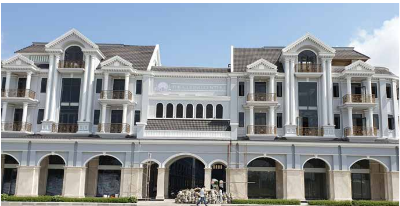
A BUILDING WHERE NITTO TAPES WERE APPLIED
