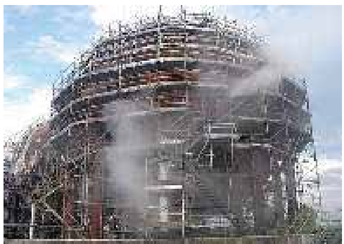
PAINT 3 VCM TANKS – TPC VINA
