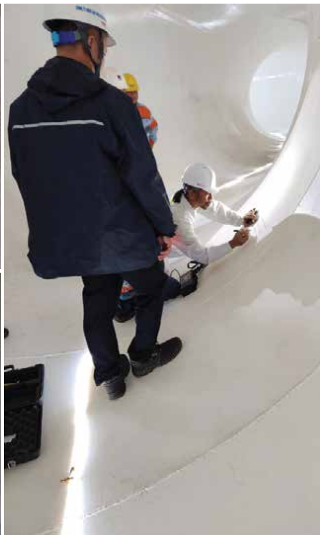
PAINTED THE INSIDE OF SEAWATER PIPELINE – VUNG ANG THERMAL POWER PLANT
